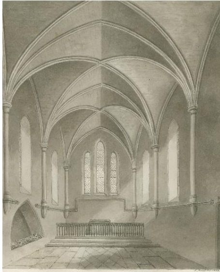
Figure 14. The chancel after the rebuilding of 1845. (William Salt library, used with permission)
