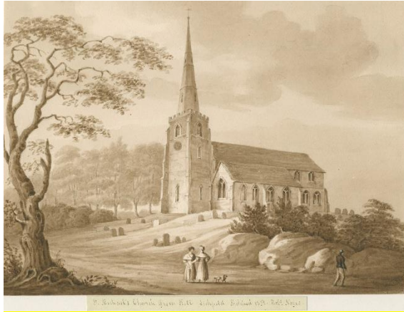
Figure 11. The church from the south in 1833 (William Salt library, used with permission)
